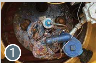
Regular Unleaded Without Sump-Dri Installed
